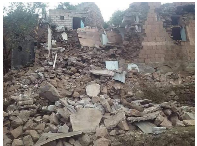
Figure 6: landslides destroyed some houses in two villages at Al-Sadah ( https://almawqeaqpost.net.2019 )
